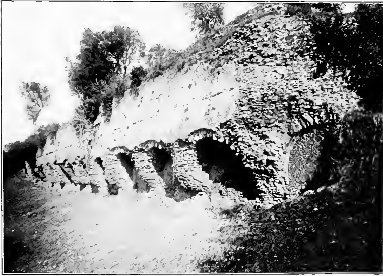
The middle terrace of the villa of Mæcenas on the Carciano road. (From a photograph by Dr. Thomas Ashby)
